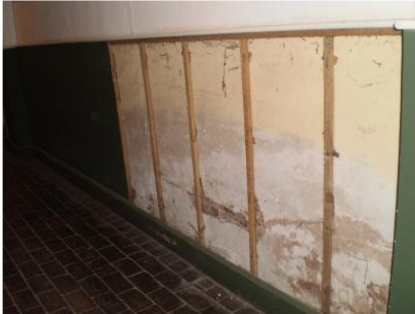
A section of the north wall of B6 opened-up to inform the capital works ( Author )
