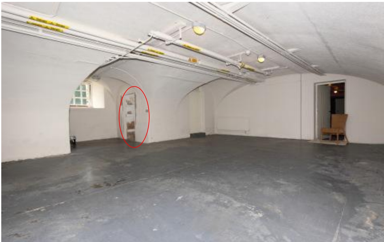
B31 looking NE and showing the cupboard in the thickness of the return wall of the NW bay of the 17 th century house ( Robert Thrift )
