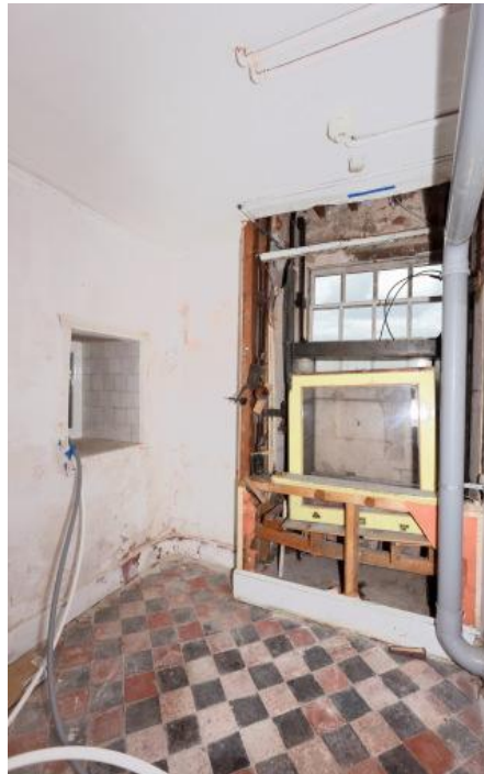
Northern end of B30 showing remains of dumb waiter and hatch on left into B28 ( Robert Thrift )
