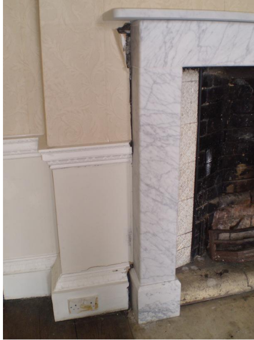
The replacement chimneypiece on the north wall of F2, showing where it has been 'let-in' (Author)
