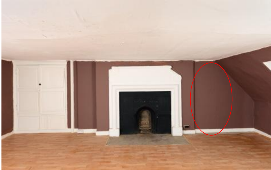
S6 looking east, showing the c.1640 chimneypiece and the location of the former connection with S3. ( Robert Thrift )
