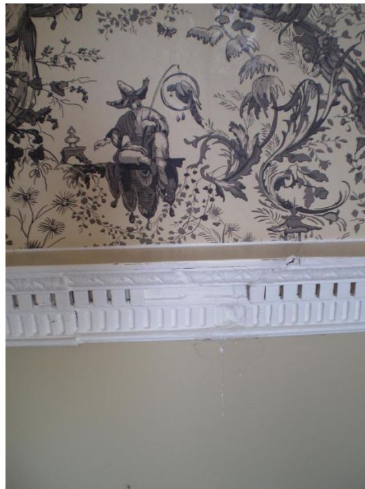
Close-up of break in dado rail giving clue to former opening in NW corner of room. Note modern Chinese wallpaper (Author)
