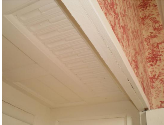
Detail of the re-used Jacobean panelling on the lintel of the jib door/cupboard ( Author )
