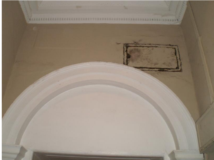
Soot door above archway in first floor corridor (F4) opened-up during flue works in 2010 ( Author )
