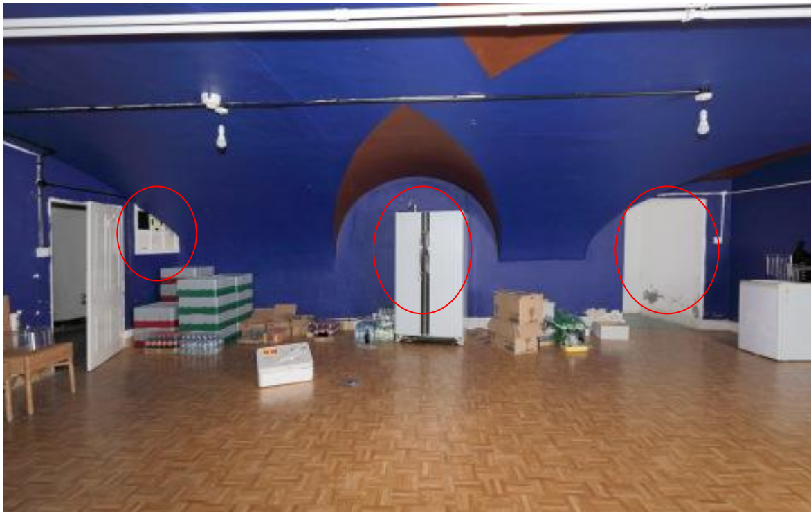
B17 looking north, indicating (middle & right) 2 blocked openings onto B6 corridor and (left) internal window on west wall ( Robert Thrift )
