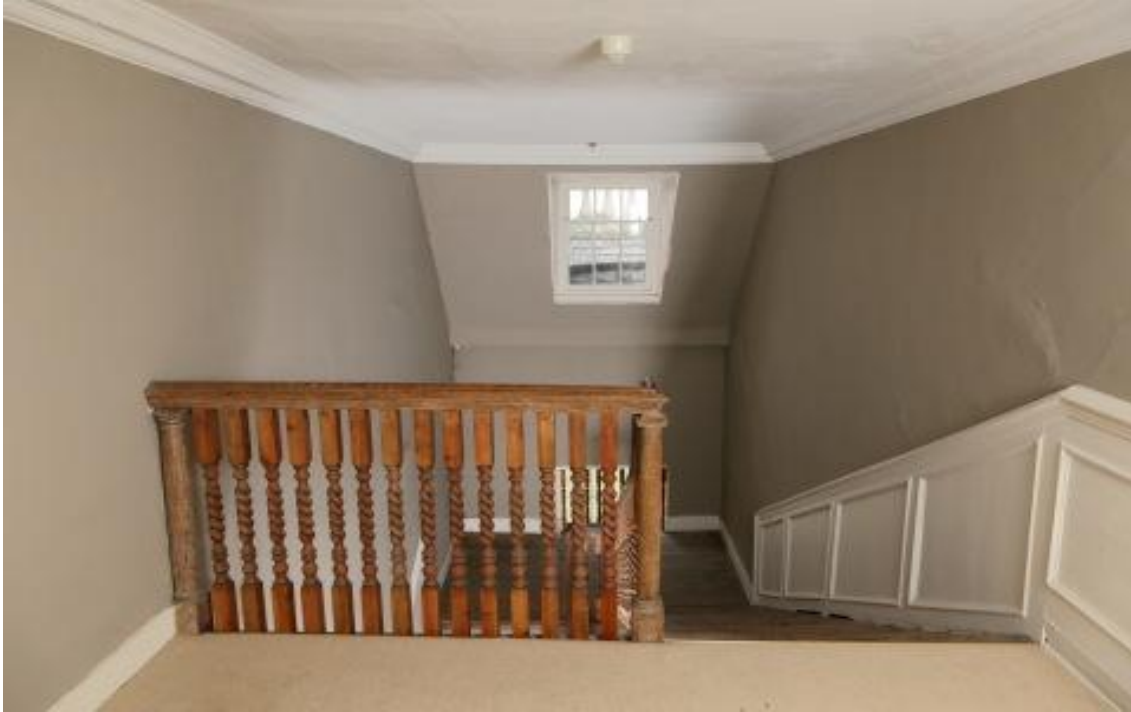
The second floor landing of the back staircase, showing original newel posts but replacement balusters, and the dado panelling on this section ( Robert Thrift )
