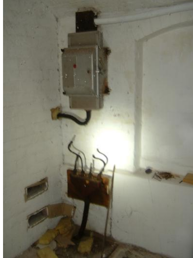
Redundant electricity intake in B20 ( Author )
