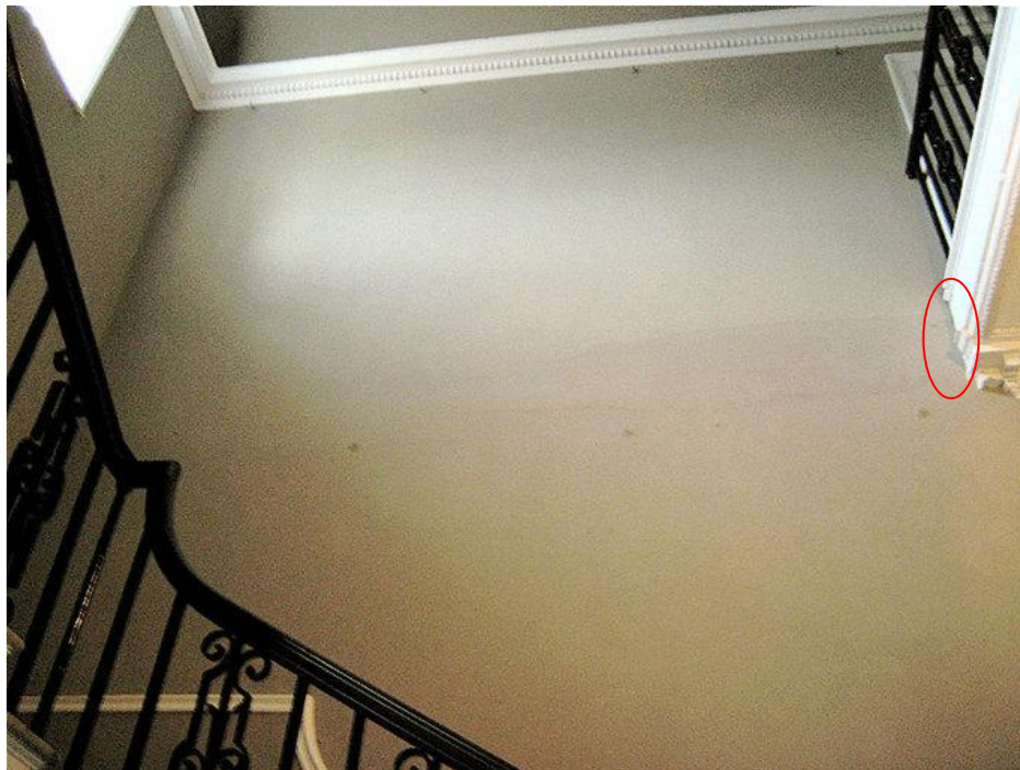
Image of top of main stairs showing post-1750s location of The Great Horse painting and indicating where the top-landing moulding was cut away to accommodate it (Author)
