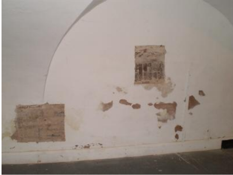
Opened-up section on north wall of B21 revealing what appears to be a blocked historic fireplace ( Author )
