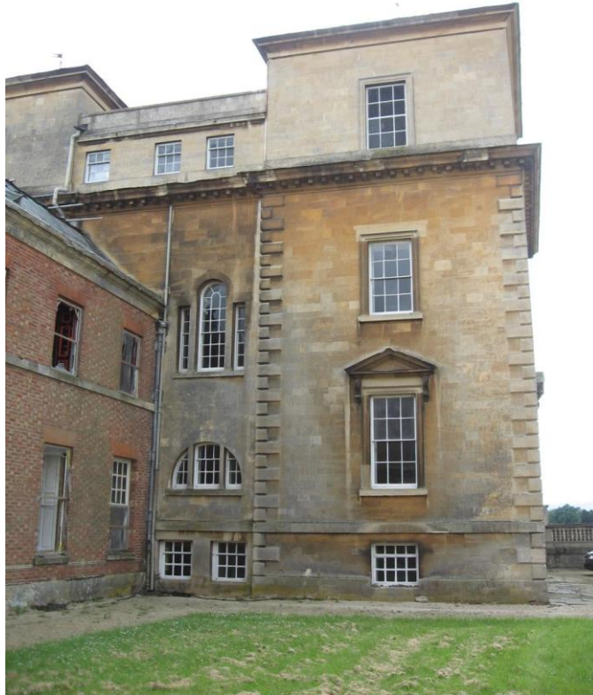
East elevation showing unsatisfactory off-set nature of main staircase due to the abutting Red Wing ( Author )
