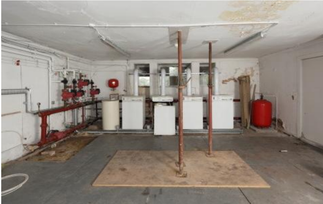
B15 looking south showing the boilers and the propped ceiling with the Library above. Note blocked opening to B17 on the right. ( Robert Thrift )
