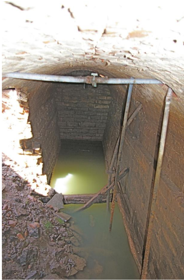
18 th century underground water chamber to the SE of the Red Wing ( Jeremy Milln )
