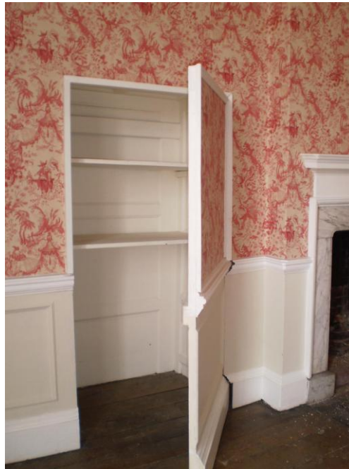
The jib door on the west wall in S3 originally leading to S6 but now forming a cupboard. ( Robert Thrift )
