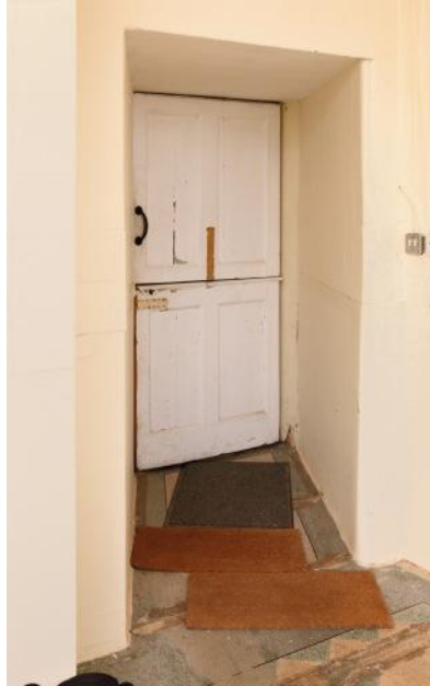
Early 17 th century modified door to B27 and diagonal passage through thickness of original external west wall ( Robert Thrift )
