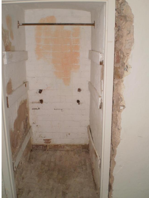
The cupboard in B31 within the thickness of the earlier wall. Note the narrow early bricks on the floor and the blue lias stone to the right of the door frame ( Author )
