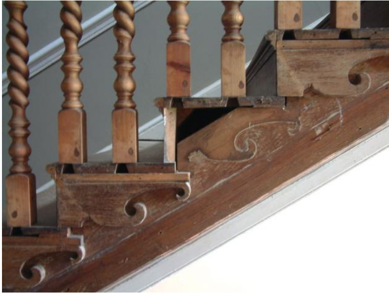
Current side view of the backstairs, showing the modern balusters and missing string detail ( Author )
