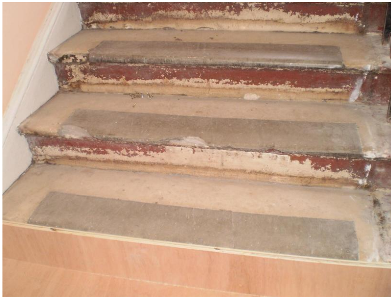
The lower reaches of the Backstairs being covered with plywood in 2009 for H&S reasons, showing the heavily repaired stone treads ( Author )
