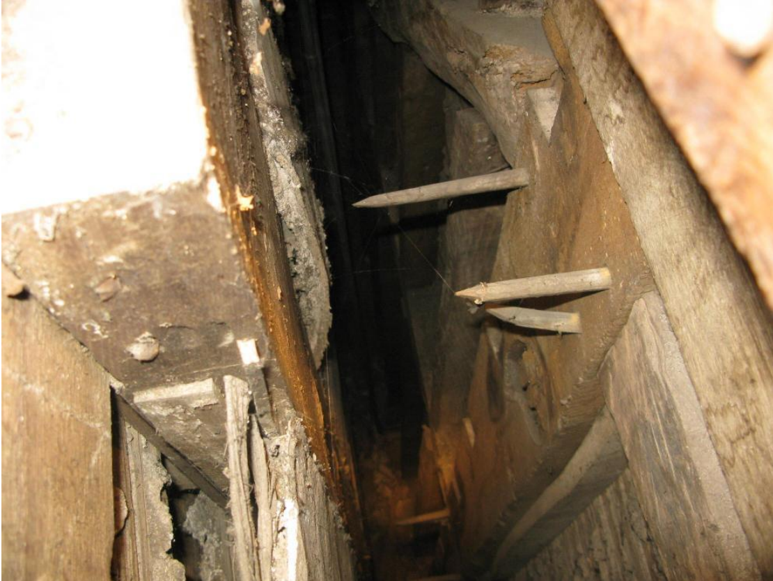
The gap between the wall at the back of the alcove in F8 and that of the Saloon descending to ground floor level. Note the large oak pegs in the timber-framed construction ( Author )
