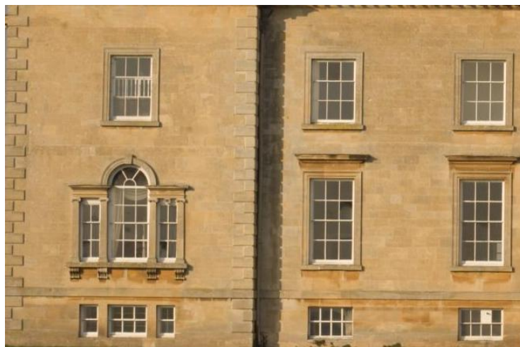
Detail of south elevation showing mis-alignment of Venetian windows on ground floor (NTPL)
