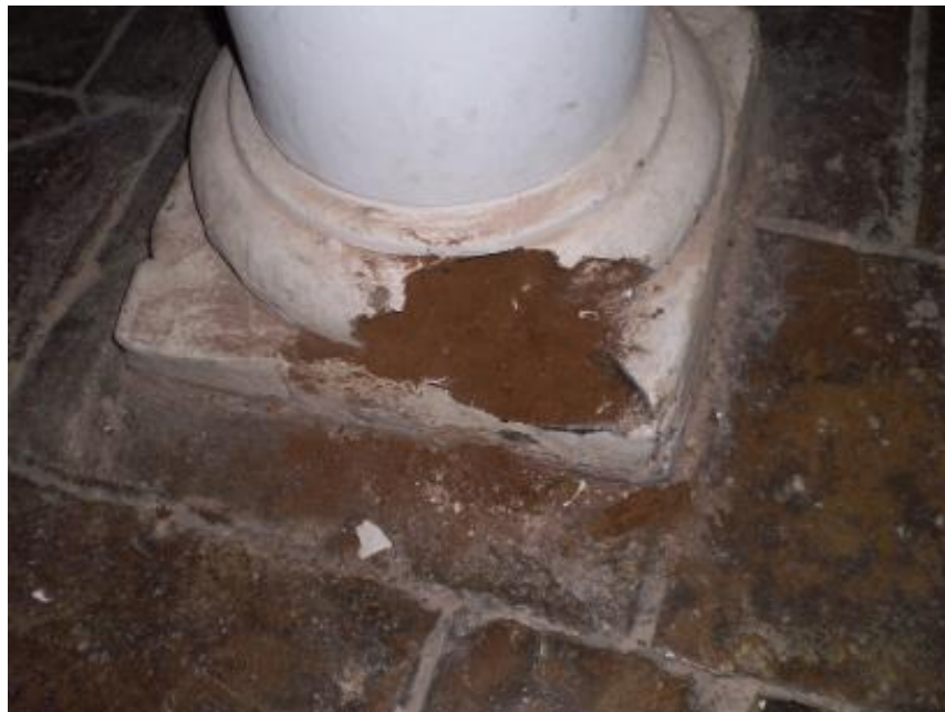
Rotting to base of column in B10 ( Author )
