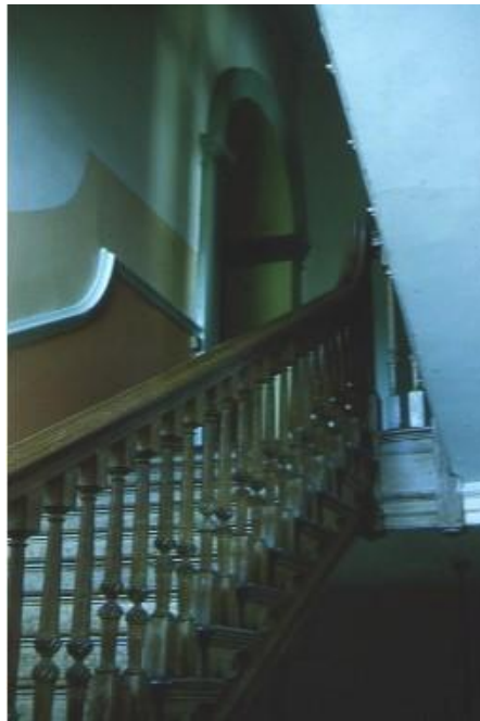
The backstairs rising to first floor level, showing the original balusters in place during the school's occupation. Note the dado paint treatment. (Leonard Edwards)
