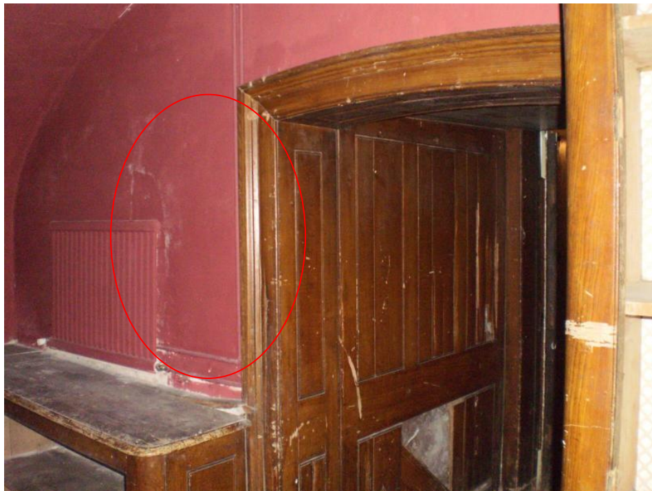
Detail of east wall of B14 and passage to B13 indicating where the ghost of a possible 17th century fireplace can be seen ( Author )
