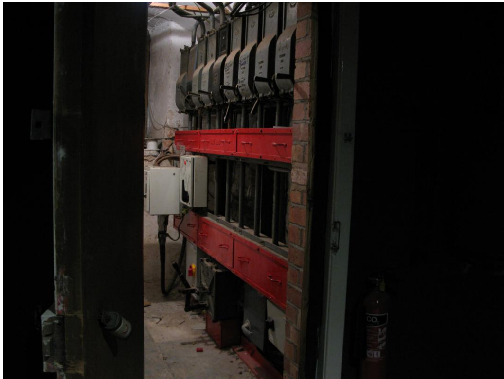
The surviving 1930s switchgear in B4 ( Malcom James )
