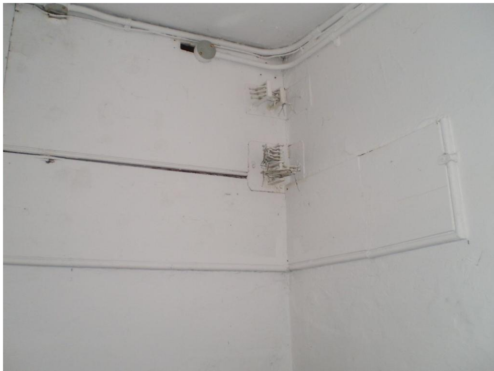
The bell board in B10 today, bereft of its bells and name plates but retaining the bell-wire hinges (Author)
